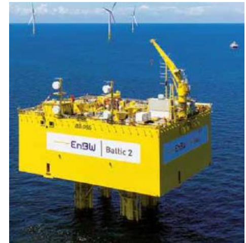
Baltic 2 Platform: Existing and already operating. Connecting the Baltic 2 wind park to the German onshore grid.
