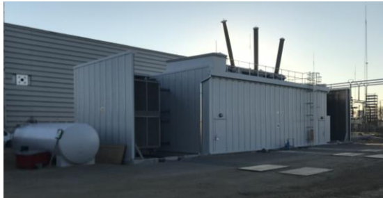
Transformer and shunt reactor hall
