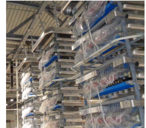
Valves assembled in valve hall
